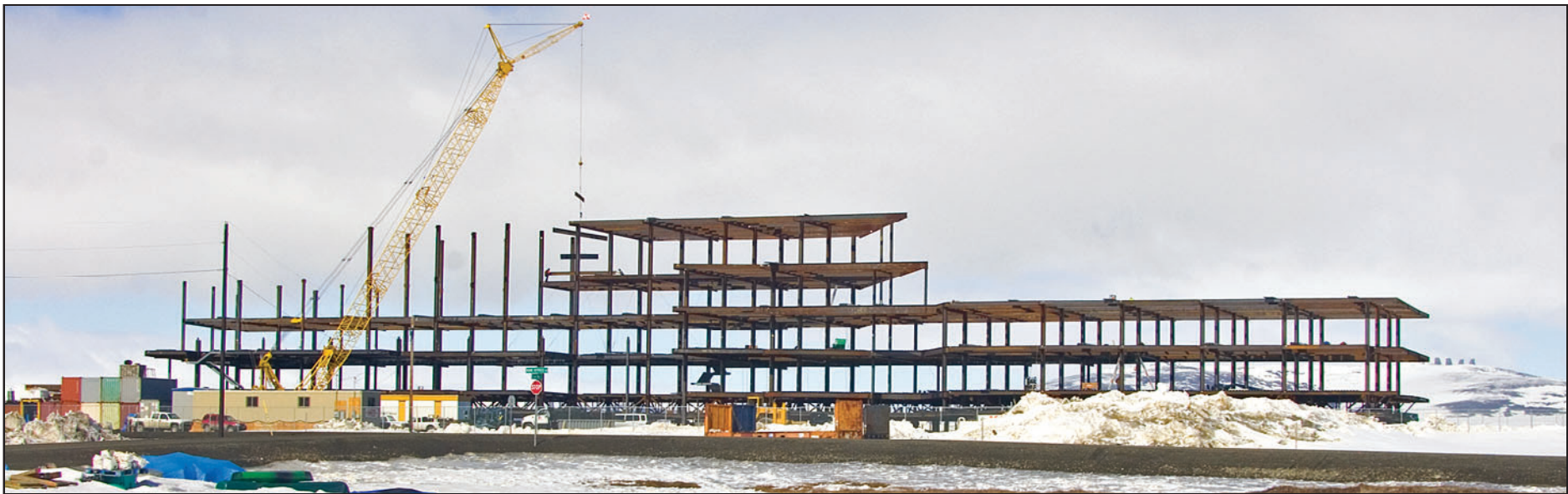
CHANGING LANDSCAPE—Norton Sound Health Corp.'s new hospital starts to take shape off of the Nome Bypass Road May 3.
